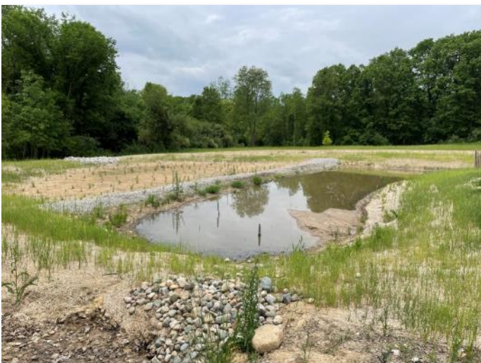
Rain garden to process rainwater from the parking lot on June 1, 2022. Area with standing water is the sediment forebay.
